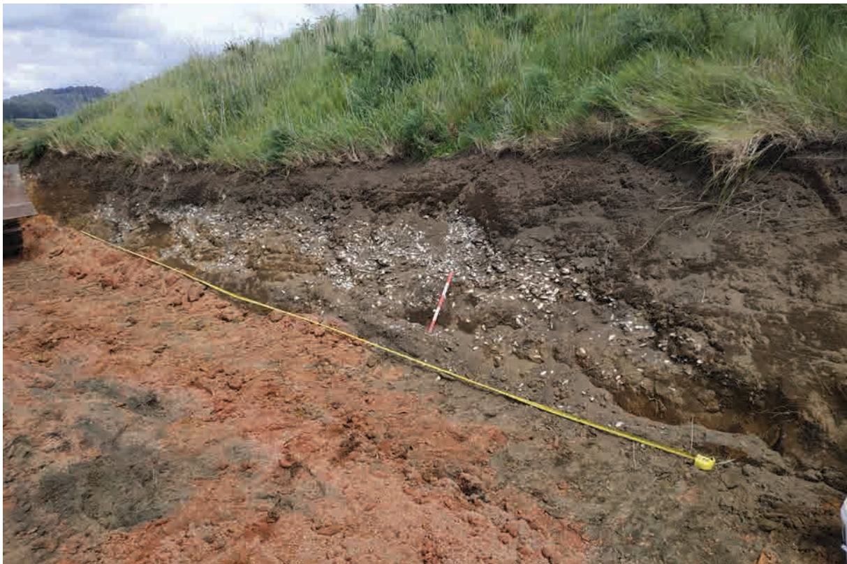
Figure 26. T11/2850 exposed in the access track cut.
